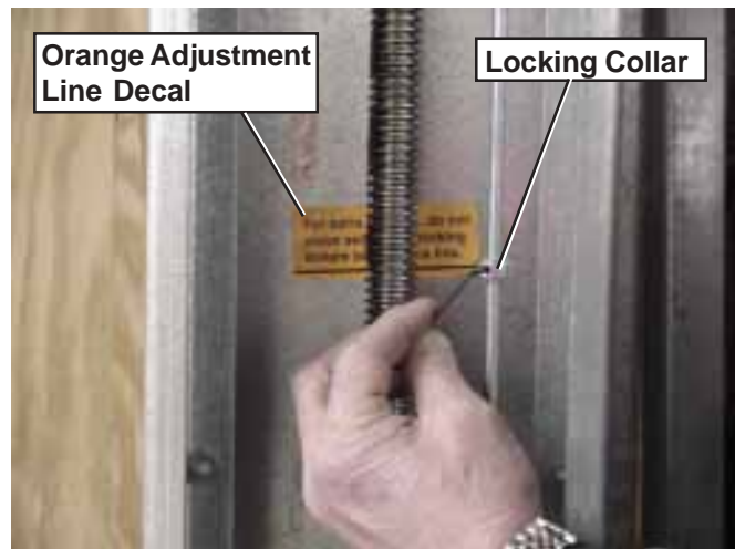
Photo 4 - Align locking collars.
