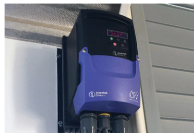
The Optidrive provides precise motor control and energy savings using the custom programs for each Commander fan.
