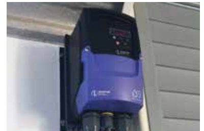
The Optidrive provides precise motor control and energy savings using the custom programs for each Commander fan.
