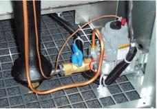
MANUAL MODULATING VALVE The manual modulating valve allows the pilot heater to be adjusted from 150,000 to 250,000 BTU to
