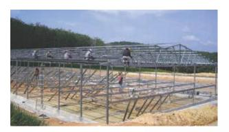
For certain applications, we offer traditional welded steel tube roof trusses. All C-Lines trusses are precision cut and welded and strong enough to suspend all necessary husbandry equipment.
