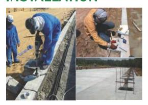
A lighter frame means a lighter concrete base. Each post of the structure stands on a solid concrete block. C-Lines ensures that these concrete blocks adhere fully to local legal codes. The concrete and fast acting chemical anchorage used ensures that Evolution® structures are quickly built and most importantly, strong.
