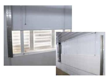
Actuated sidewall inlets are field cut to length on site allowing your system to be customized for a perfect fit every time.
